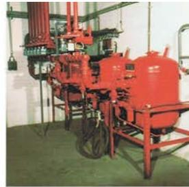
Stationary powder extinguishing system with temperature sensor
